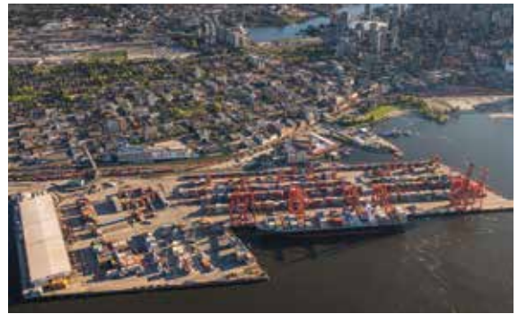
The Centerm Expansion Project on the south shore of the Vancouver harbour
