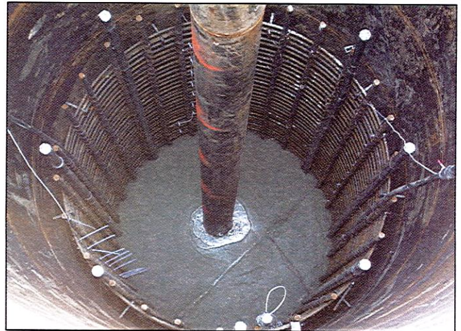
Figure 1 - Use of a tremie pipe in pouring a reinforced CIP pile.
