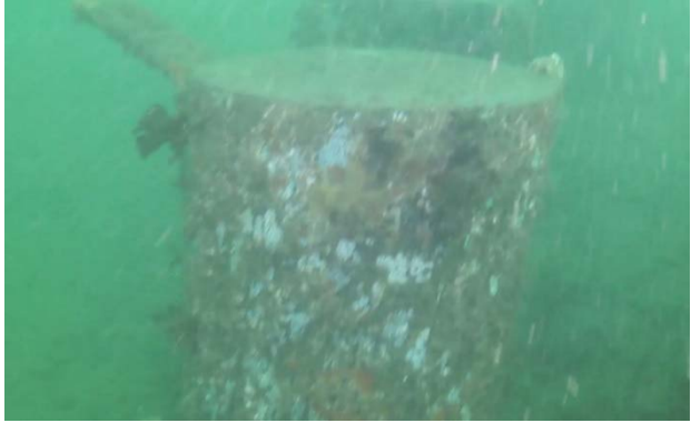
Photo 25 Transect 4 Sawn off pier pylon near endpoint of video survey
