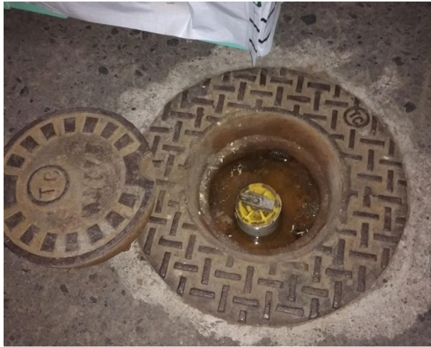
Photo 11 Monitoring well inside the storage warehouse (MW08-11).
