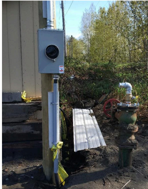
Photo 13 New upgrades to the utility pole.
