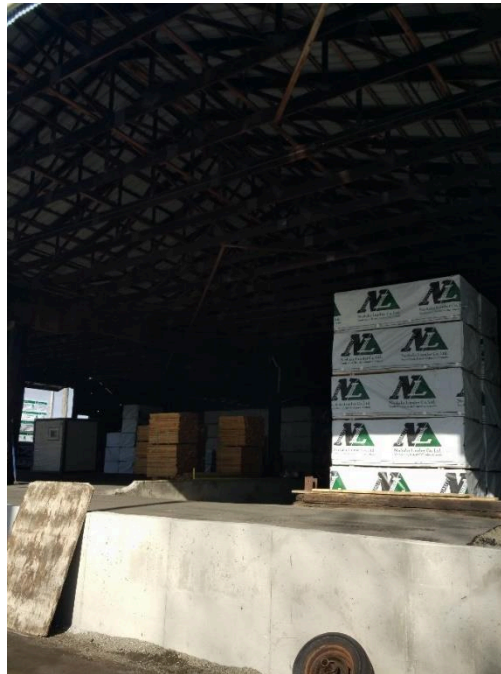
Photo 4 Open warehouse building for wood storage.
