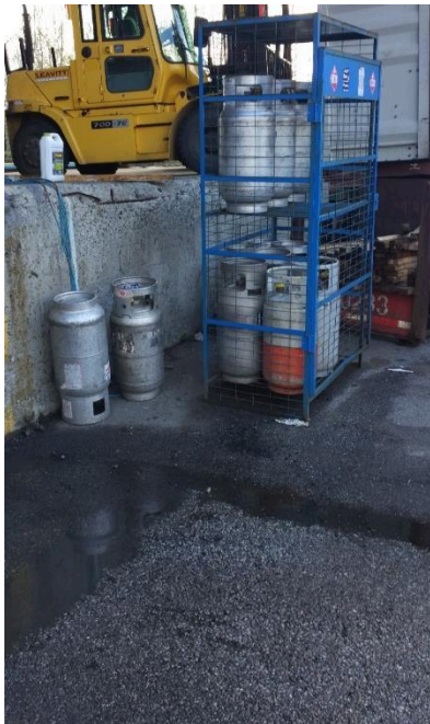
Photo 12 Propane storage inside the warehouse.
