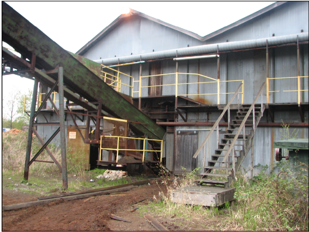
PHOTO 2: Parcel A - View of the sawmill, looking northwest.
