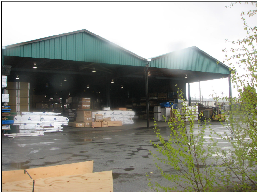
PHOTO 8: Parcel C - Looking southeast at the distribution warehouse.
