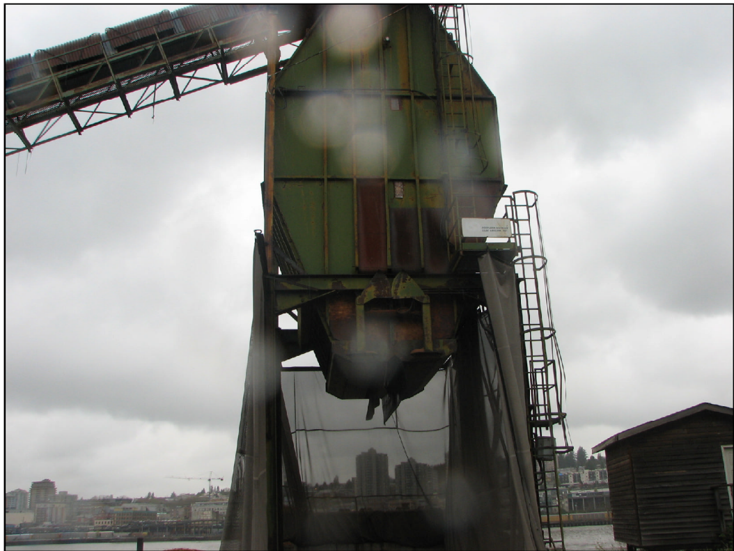
PHOTO 12: View of chip fuel bunker, off-site.
