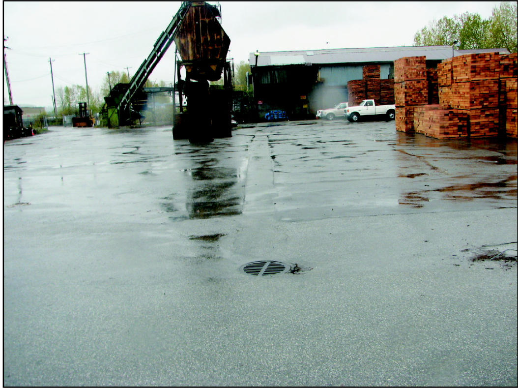
PHOTO 5: Parcel A - Looking southwest at the hog-fuel bunker.
