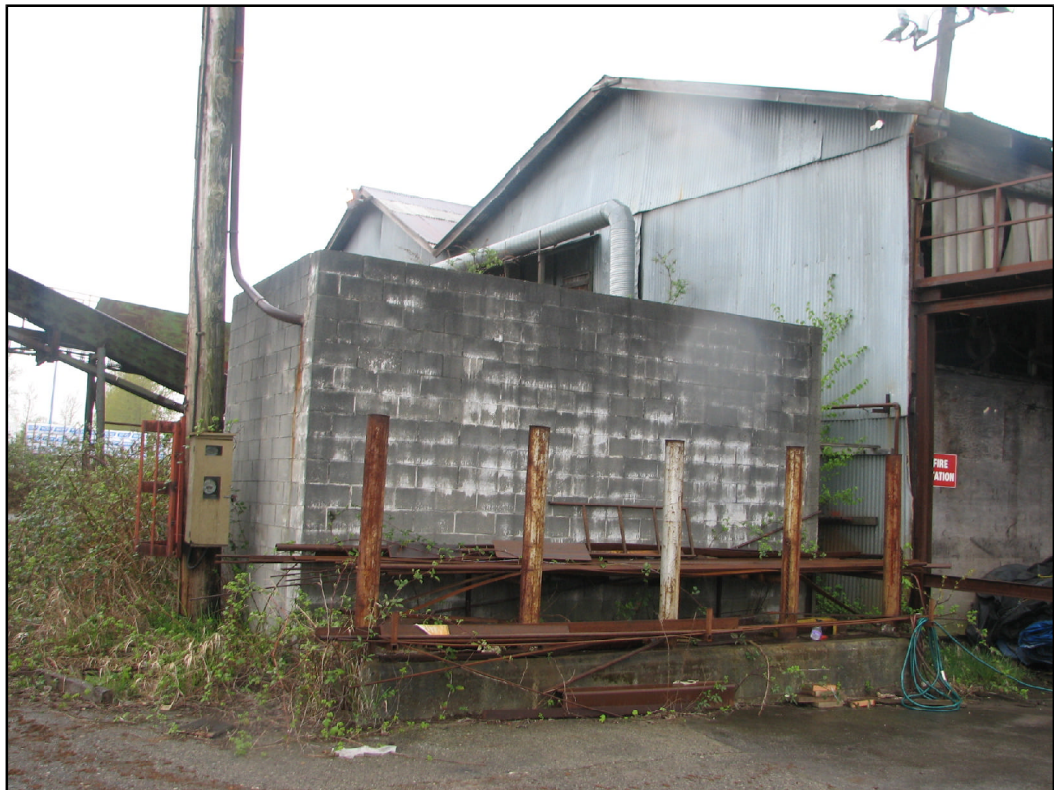
PHOTO 19: Parcel A - Mill Electrical Building.
