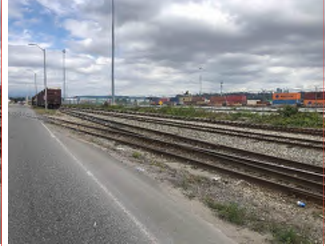
L - West Approach Drivers View Right (At Stopped Position)
