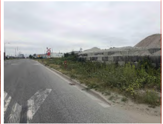
C - North Approach Drivers View Right
