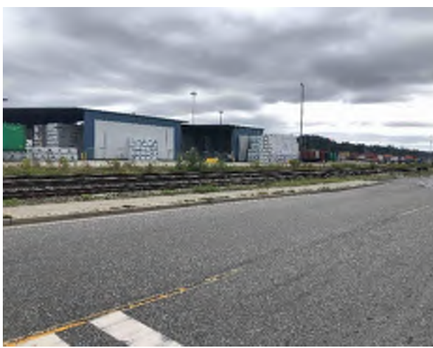
J- South Approach Drivers View Left (At Stopped Position)
