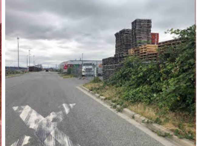
F - South Approach Drivers View Right
