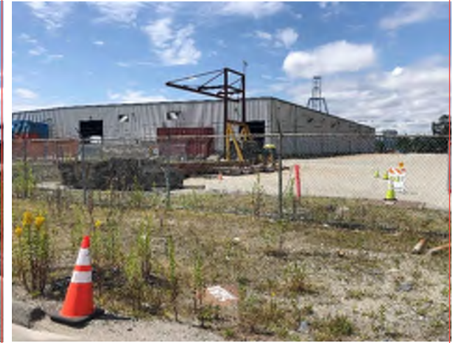
C - East Approach Drivers View Right
