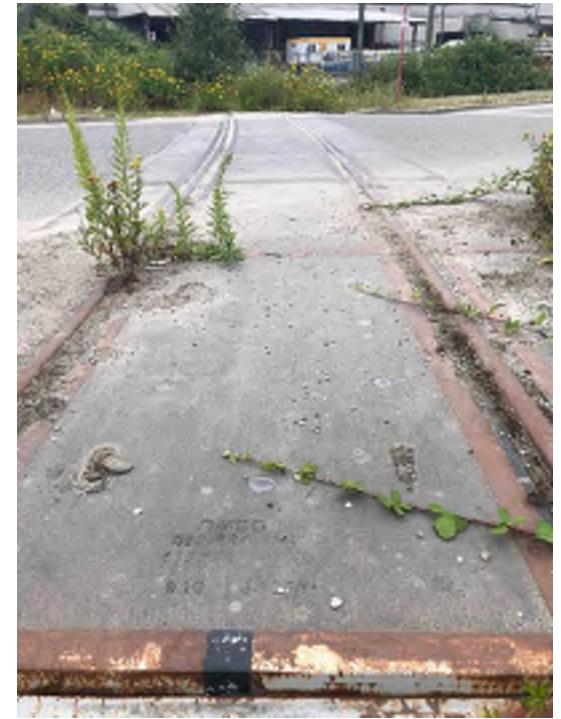
O – South Facing Crossing Surface
