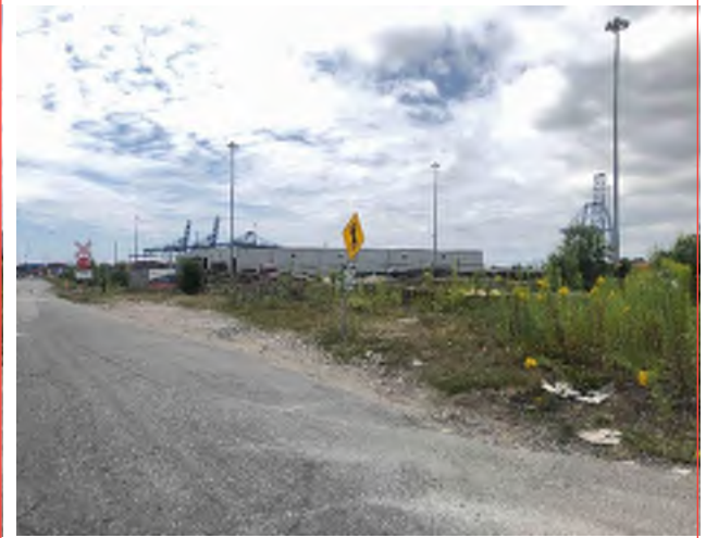
C - East Approach Drivers View Right
