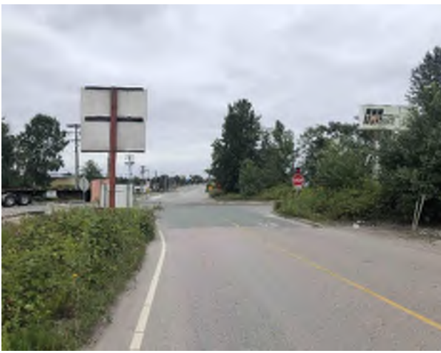
A – East Approach (South)
