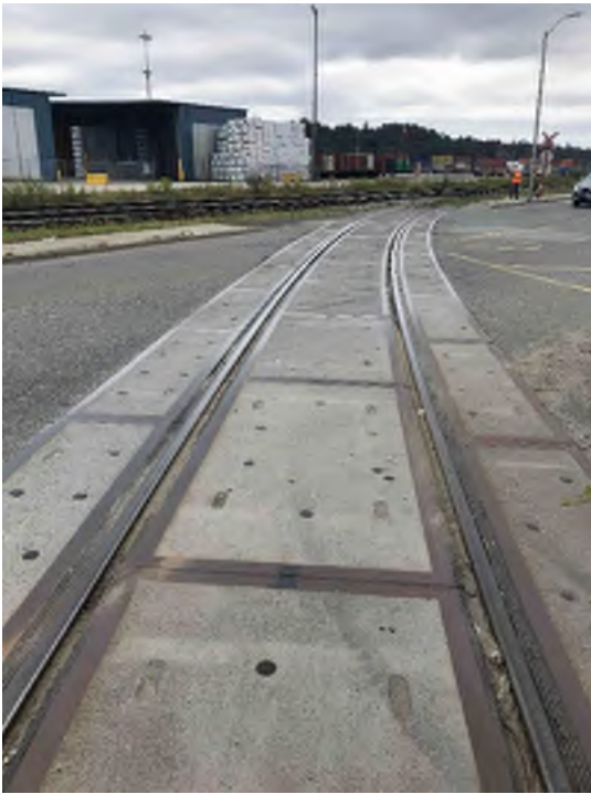
M – East Facing Crossing Surface
