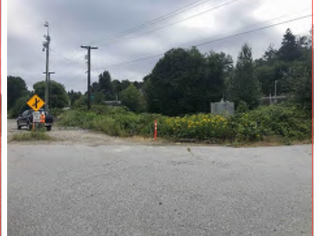
F - South Approach Drivers View Right
