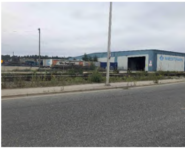
A - North Approach Drivers View Left
