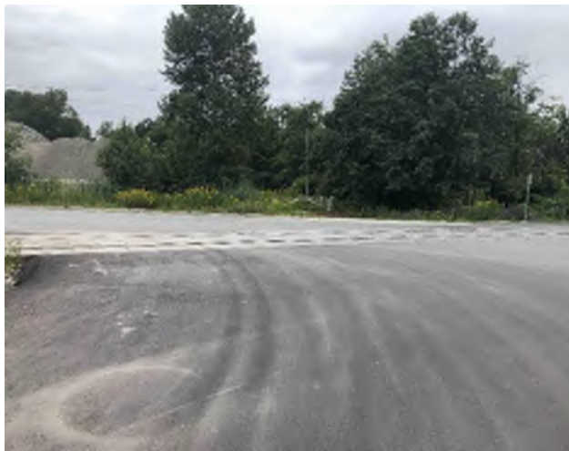
H - East Approach (At Stopped Position)
