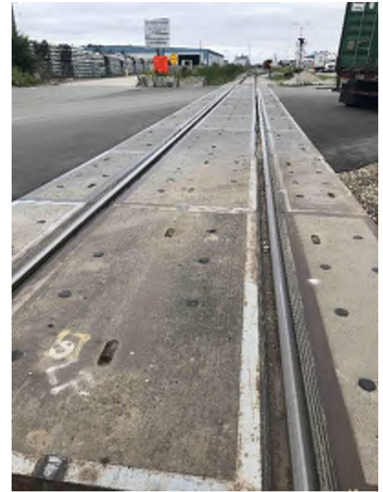
O – South Facing Crossing Surface
