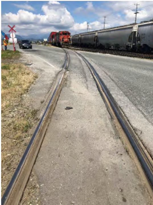
M – East Facing Crossing Surface
