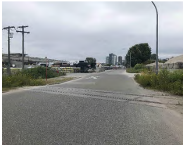
H - East Approach (At Stopped Position)
