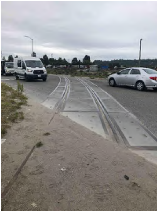
M – East Facing Crossing Surface
