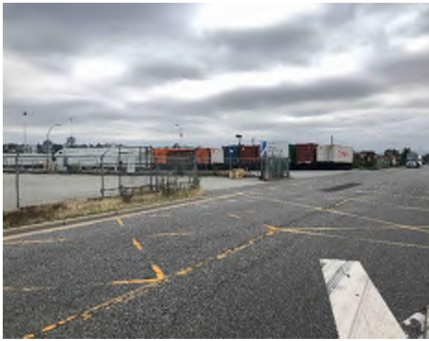
A - North Approach Drivers View Left
