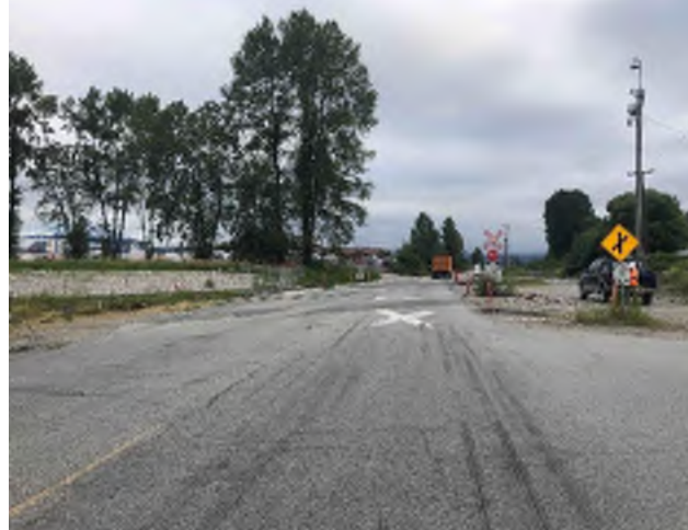
E - South Approach
