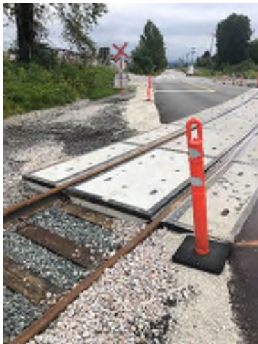
M – East Facing Crossing Surface
