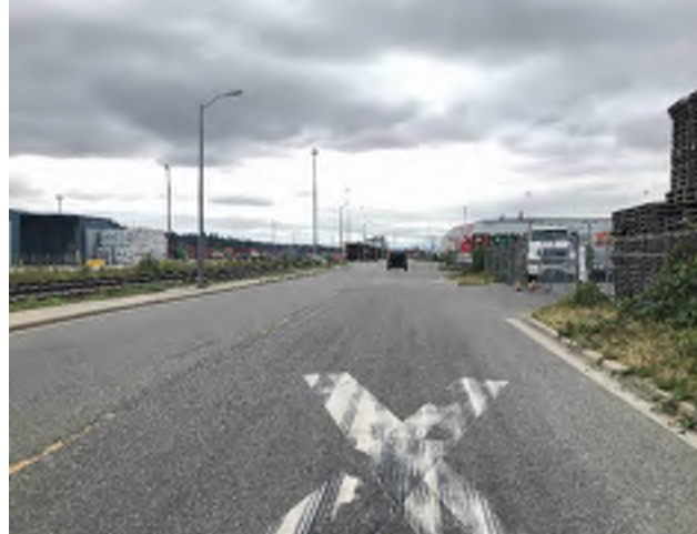
E - South Approach
