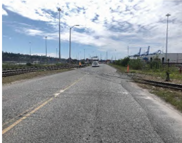
H - East Approach (At Stopped Position)
