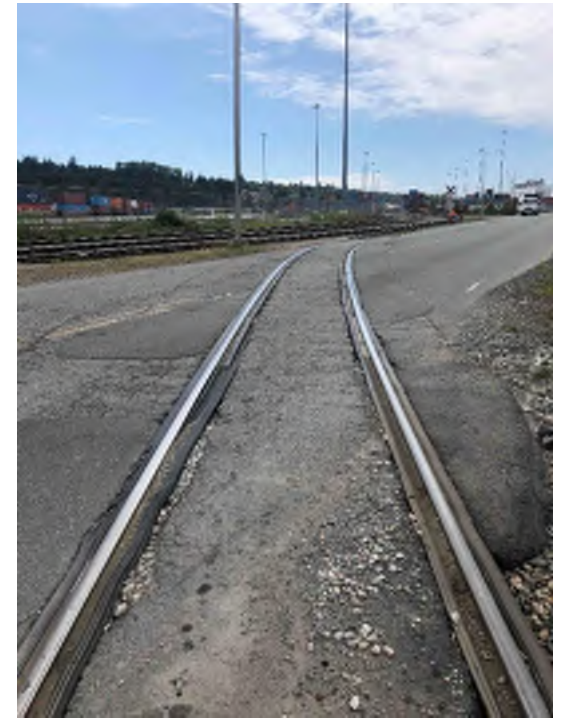
O – South Facing Crossing Surface
