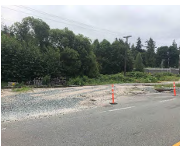
A - North Approach Drivers View Left
