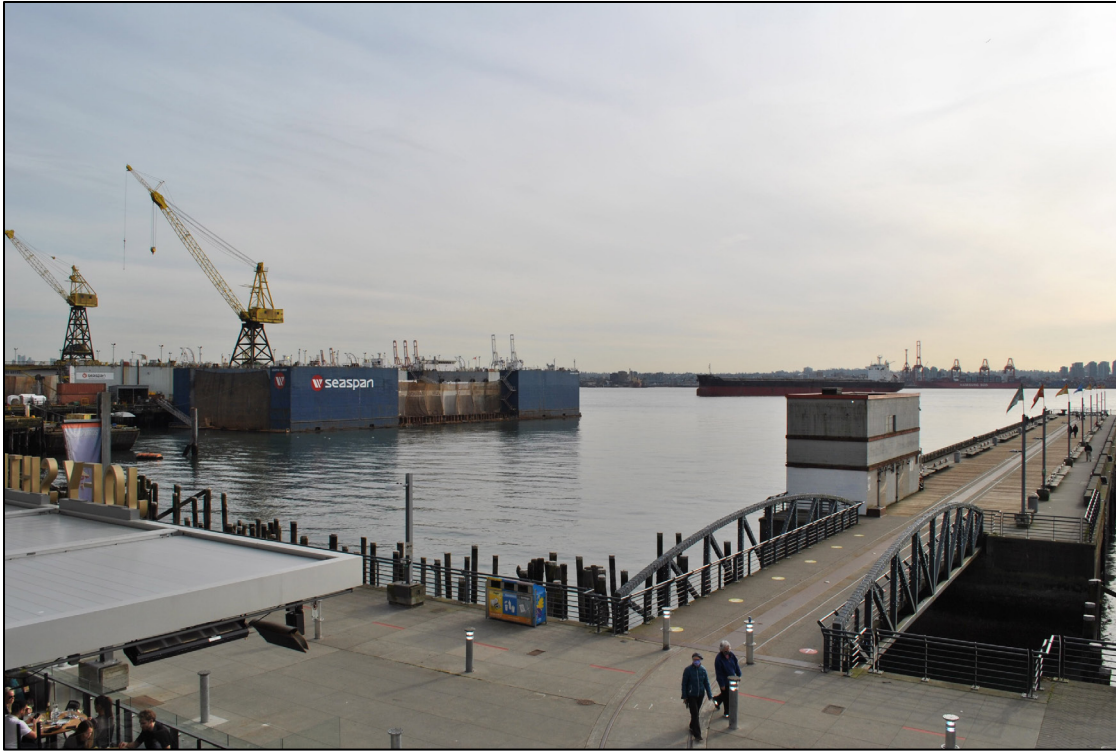
Figure A8a.9 View from Shipyard Square (west of VDC), facing south. Current (top) and proposed (bottom) drydock infrastructure. Point 2 in Figure A8a.1.
