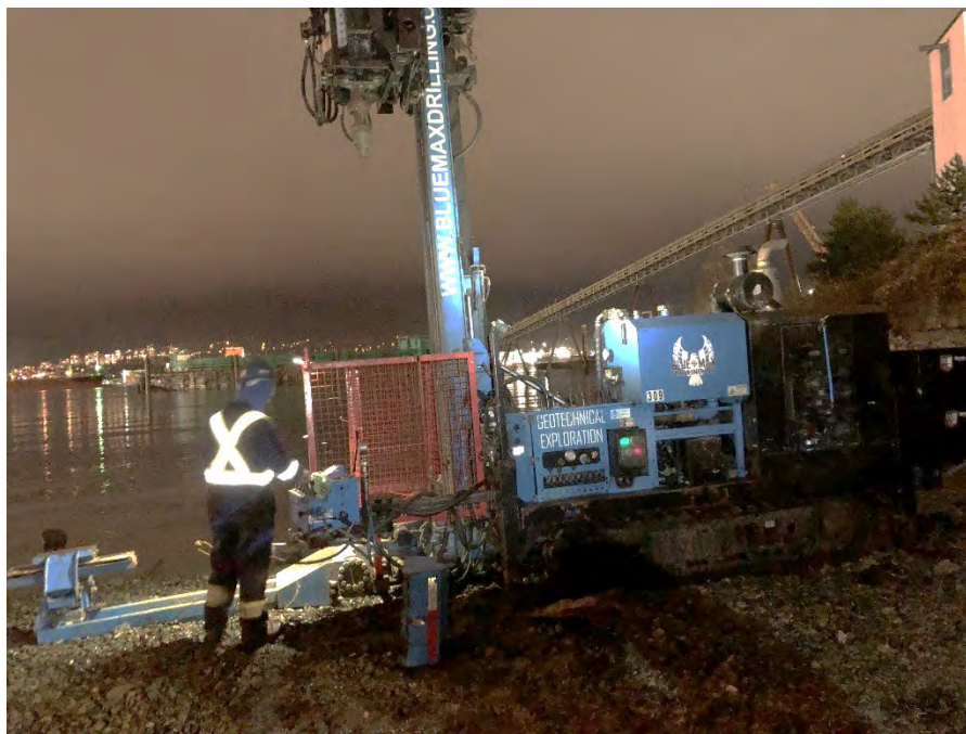
Photograph 3.2: Blue Max track-mounted sonic drill rig used for borehole drilling.
