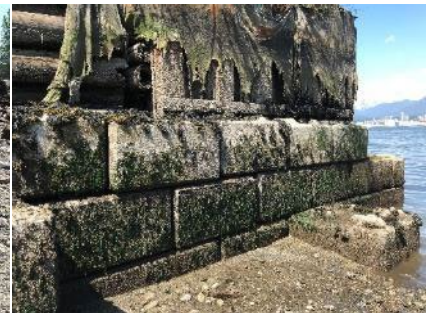
Figure 3: Concrete lock-block wall
