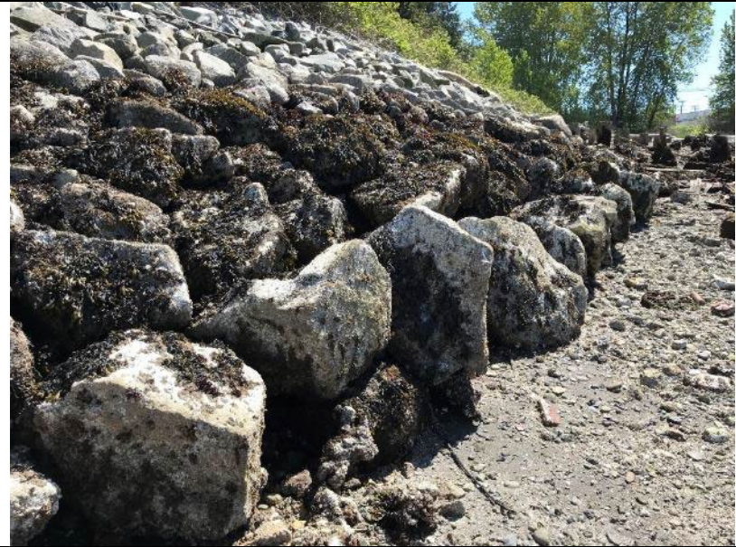
Photograph 12: Typical riprap breakwater habitat observed on-site.
