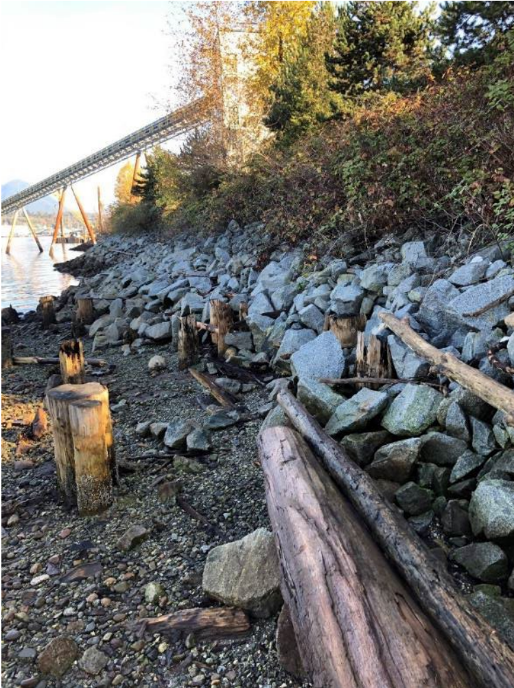
Photograph 3: Eastern Retaining Wall, facing northeast (SNC-Lavalin, October 26, 2020).
