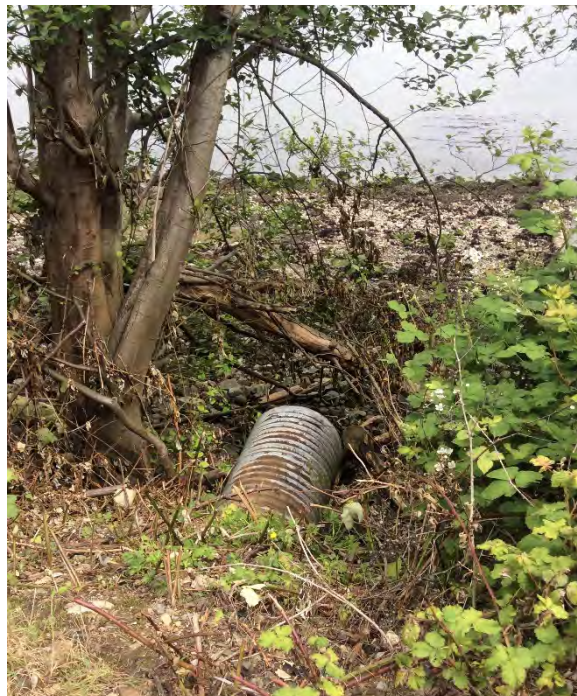
Photo 8 Culvert outlet. Photo facing north.
