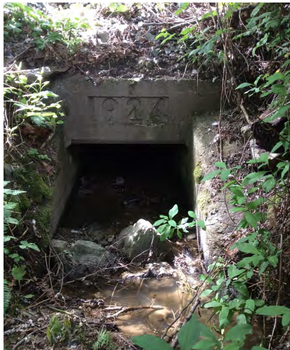
Photo 14 Concrete box culvert outlet (June 19, 2020).
