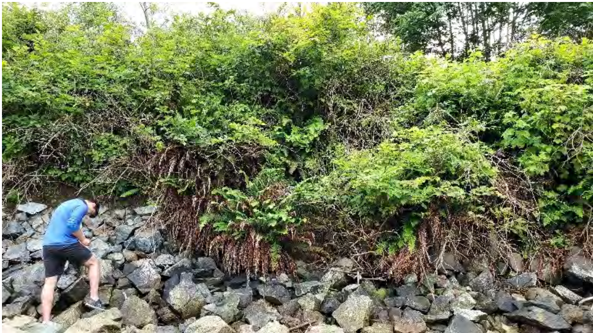
Photo 16 Representative photo of riparian stand to the east of the refinery. Photo facing south.
