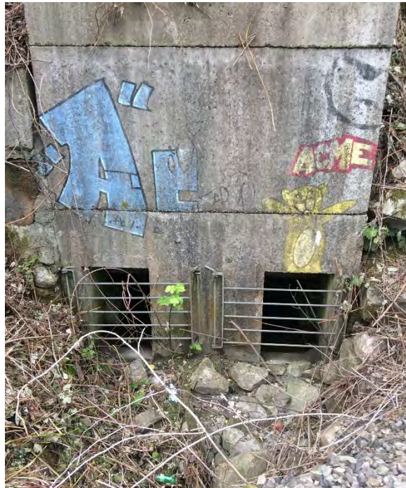
Photo 7 Looking at Structure-1 drainage conveyance structure (June 19, 2020).
