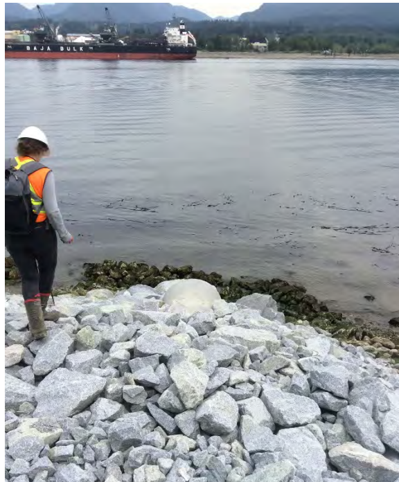
Photo 4 Crabtown Creek culvert outlet to the Burrard Inlet; facing north (June 19, 2020).
