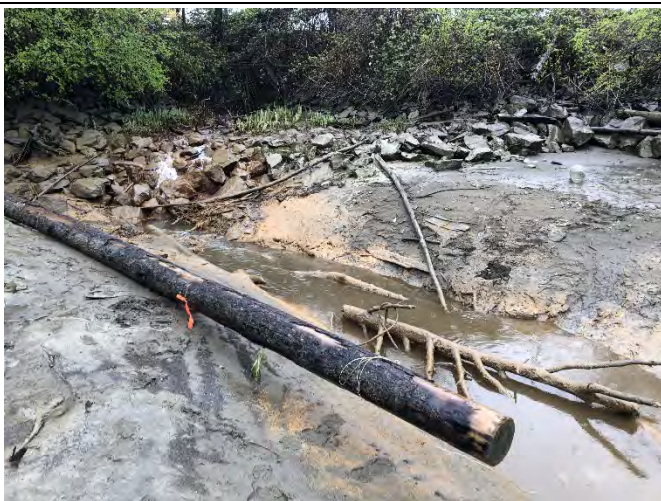
Photo 15 Outlet to backchannel facing east towards culvert and fence line. April 18, 2022.
