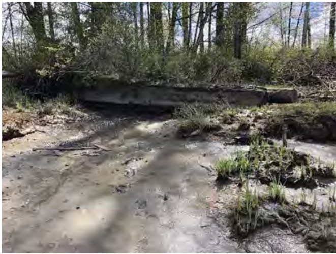
Photo 21 Outlet on shore possibly from back channel. April 19, 2022.
