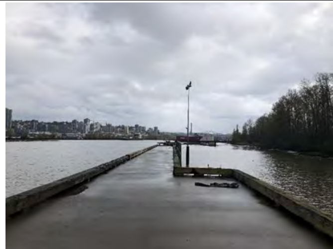
Photo 4 Facing northeast on berth 10 wharf. April 12, 2022.
