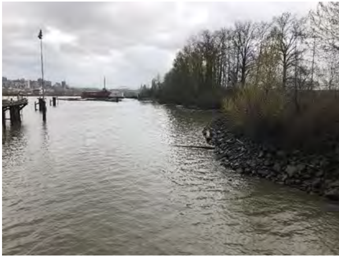
Photo 5 Facing northeast with berth 10 wharf to left, and rip rapped banks to right. April 12, 2022.
