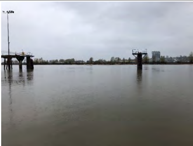
Photo 3 Location for proposed platform at berth 10, facing north from shore. April 18, 2022.
