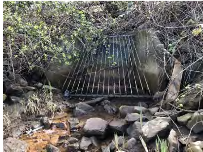
Photo 10 Debris guard on culvert outfall. April 19, 2022.
