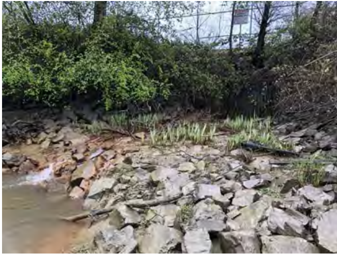
Photo 9 Culvert outfall, facing east towards fence line. April 18, 2022.
