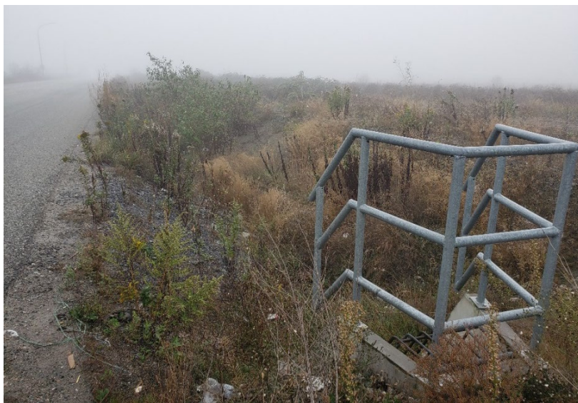
Photo 15 Ditch connecting to culvert along Portside Road
