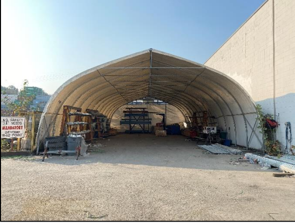
Photo 5 Anthropogenic structures on the property. No evidence of nesting birds was observed. (2022-10-18)
