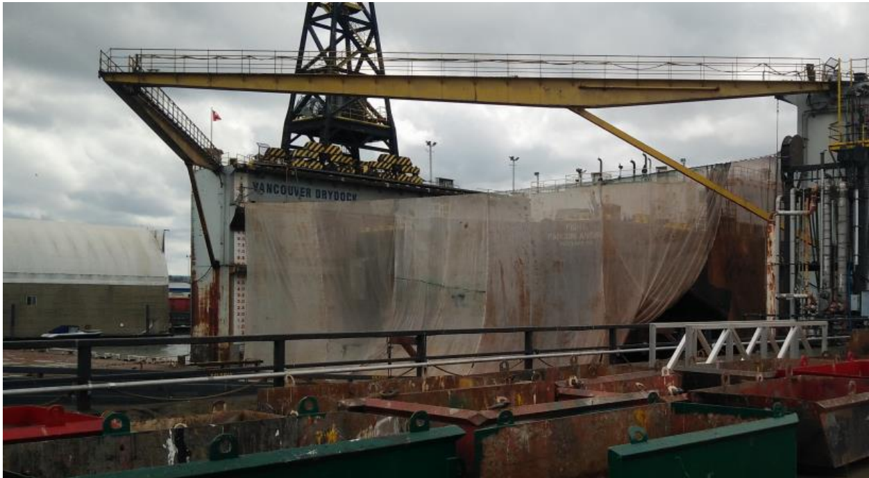
Figure 15: Existing Dust Control Curtains
