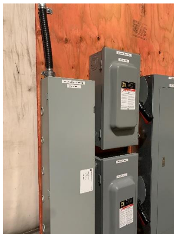
Figure 3: New distribution equipment Installed by Mott Electric East Wall Warehouse Building
