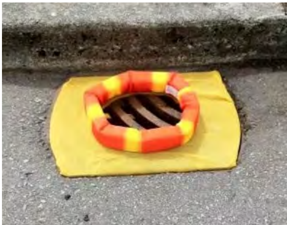
Figure 1: Catch Basin "Donut" (Photo credit: BMP Supplies)
