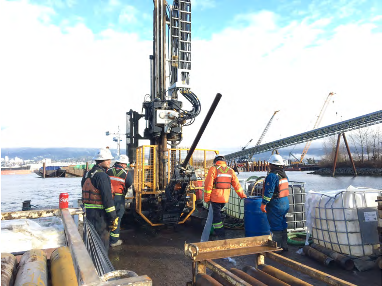
Photograph 1: Sediment investigation borehole drilling (hands-free drill rod handling and safety cage being used).
