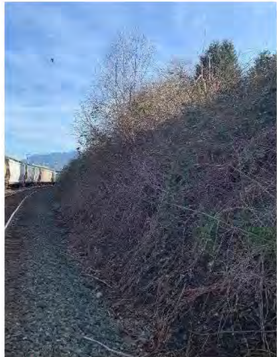
Photo 6: Himalayan blackberry growing extensively along the embankment along the south side of the CP right-of-way.
