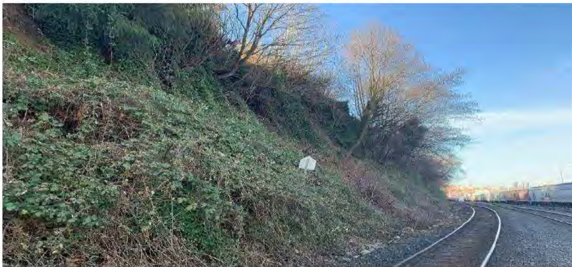
Photo 3: Typical vegetation community on the south side of the CP right-of-way adjacent to Commissioner Street comprising an understory dominated by invasive species and sporadic native and non-native tree species.
