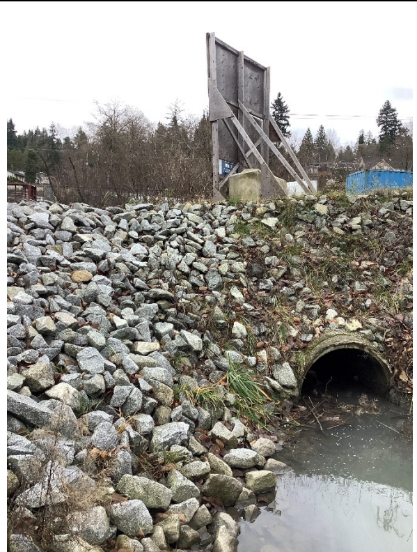
Photo 8: Site 4, looking at concrete culvert under Robson Road.
