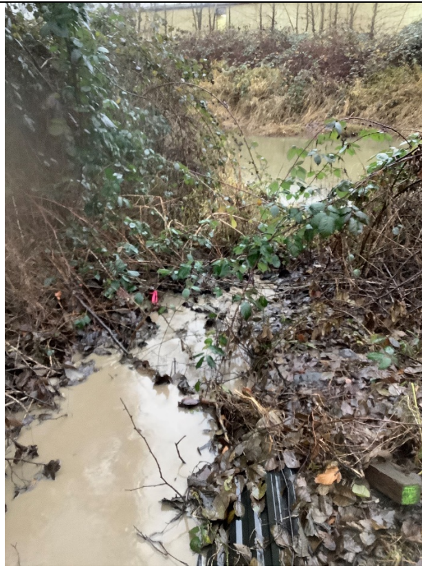
Photo 20: Site 9 and 10, looking downstream (north) at outlet to Manson Canal on the west side of Timberland Road.
