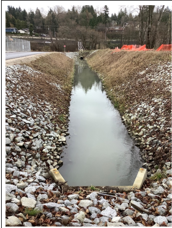
Photo 7: Site 4, drainage ditch looking east towards Robson Road.
