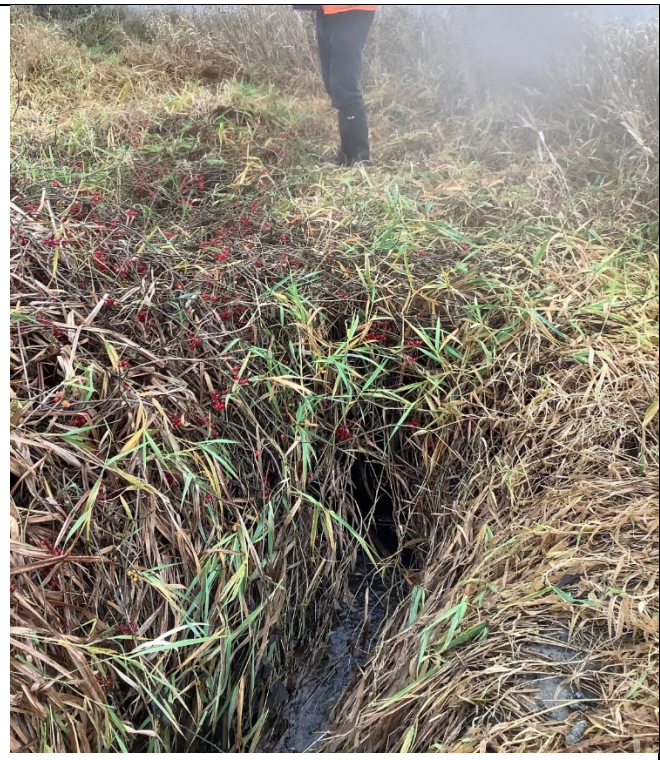
Photo 6: Site 3 Unnamed Creek looking upstream (east) towards culvert under Robson Road.
