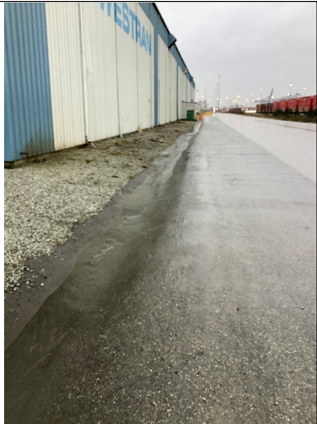
Photo 16: Site 8 looking upstream at pavement ditch collecting surface runoff.
