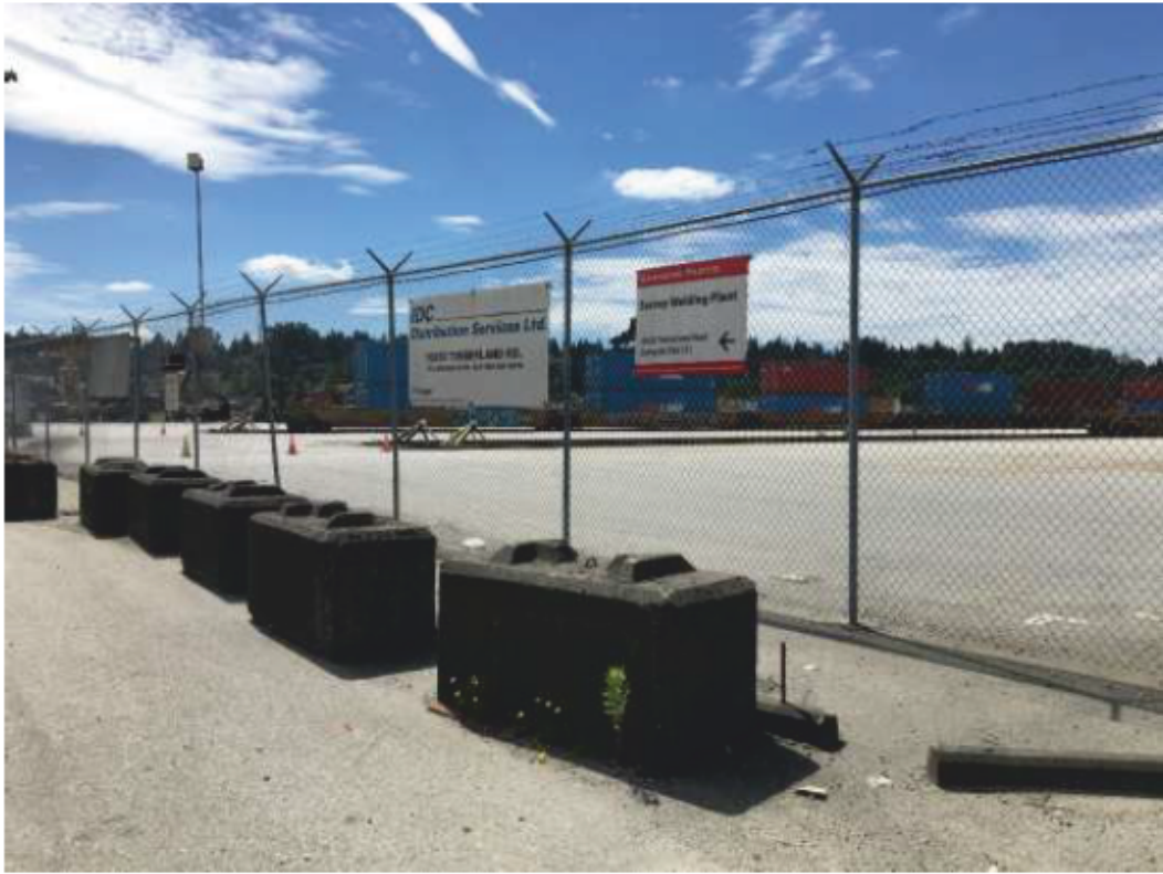
Photograph 5: 10550 Timberland Road – occupied by IDC Distribution Services Ltd.
