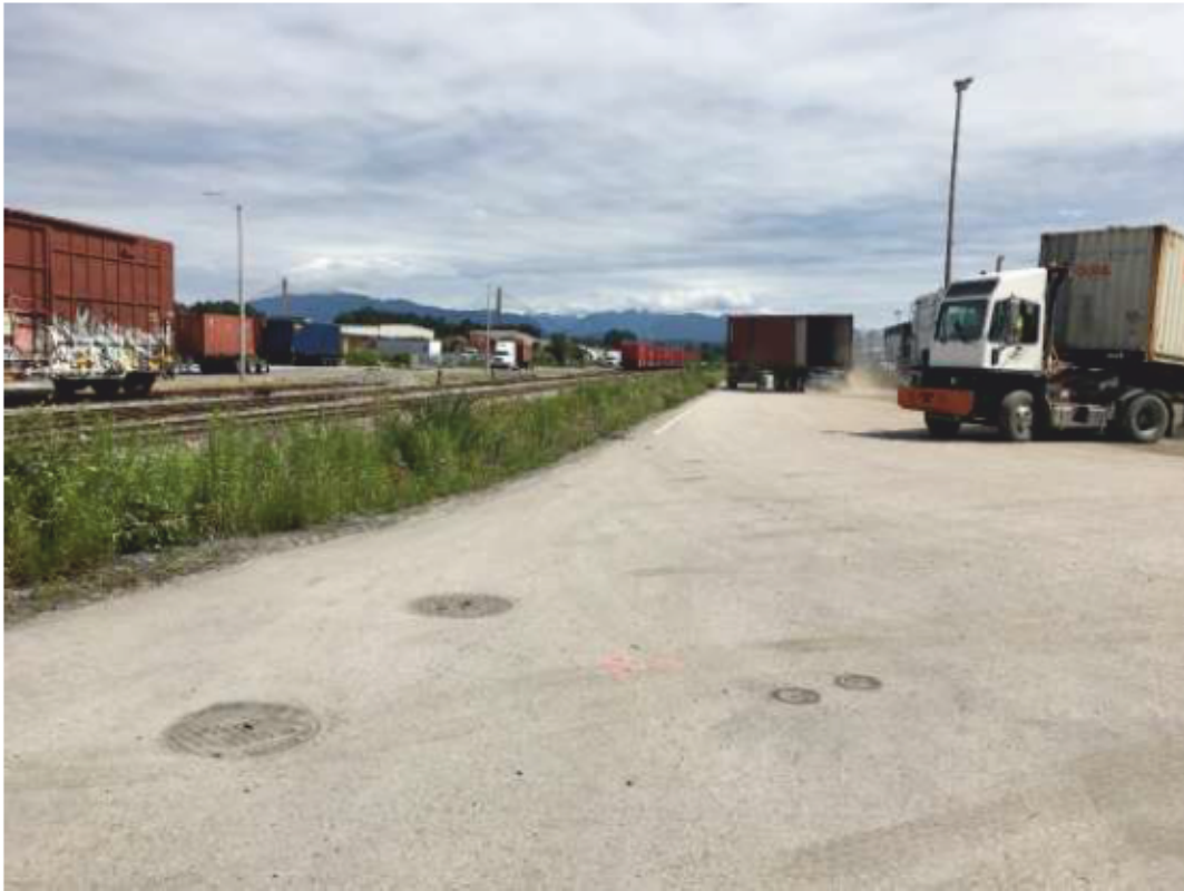
Photograph 1: View of Timberland Road looking north.
