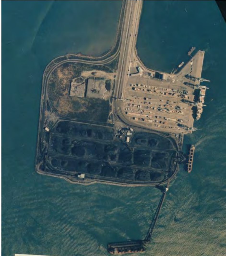
1997 – Coal Storage expanded to Pod 2 Row D, Deltaport constructed in Pod 4, Preloading in Pod 3
