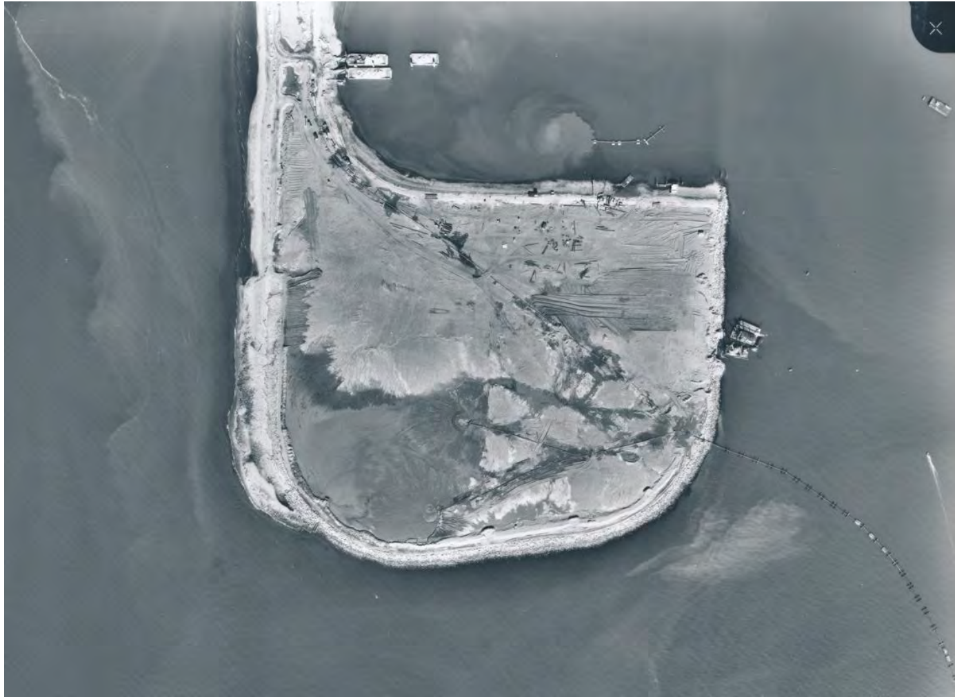
1969 – Pod 1 Fill Placement
