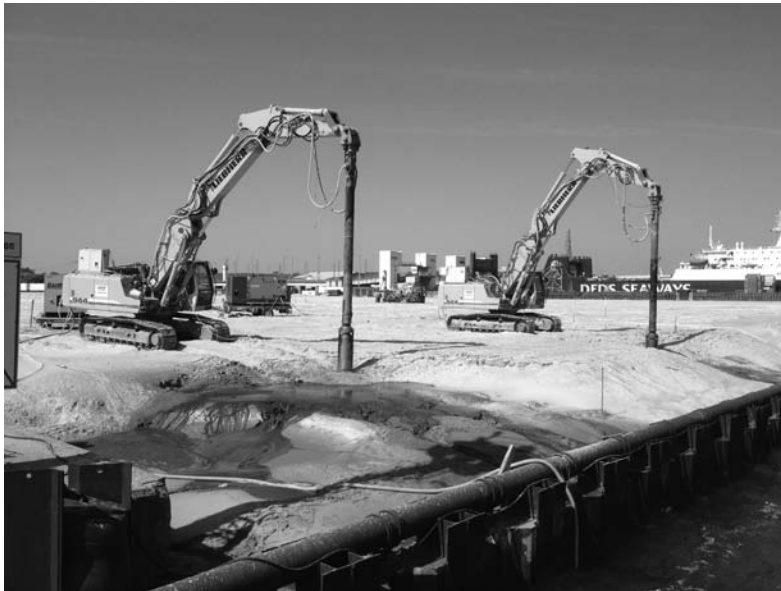
Figure 16.32 Construction of a stone column [DGI-Menard (USA).]
