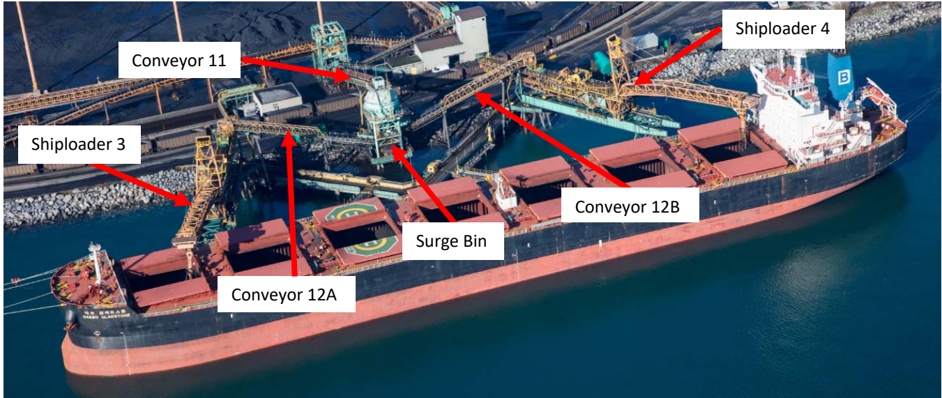
Figure 1: Existing Berth 2 Infrastructure
