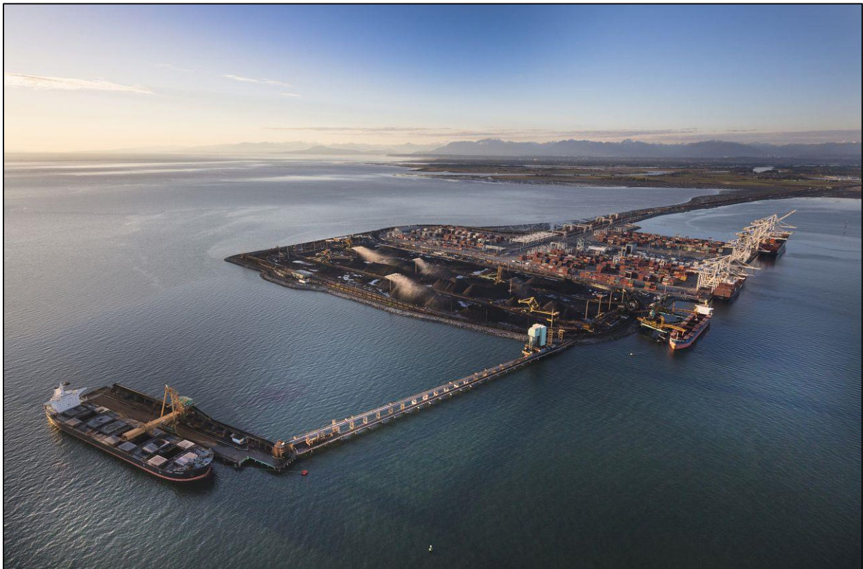
Figure 1: WTLP – Aerial View
