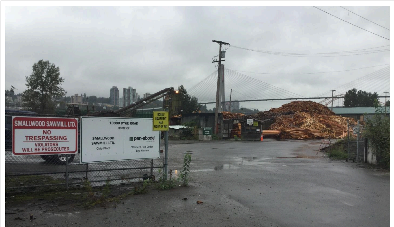
Photo 1. Front view of the Site from Dyke Road, facing northwest.
