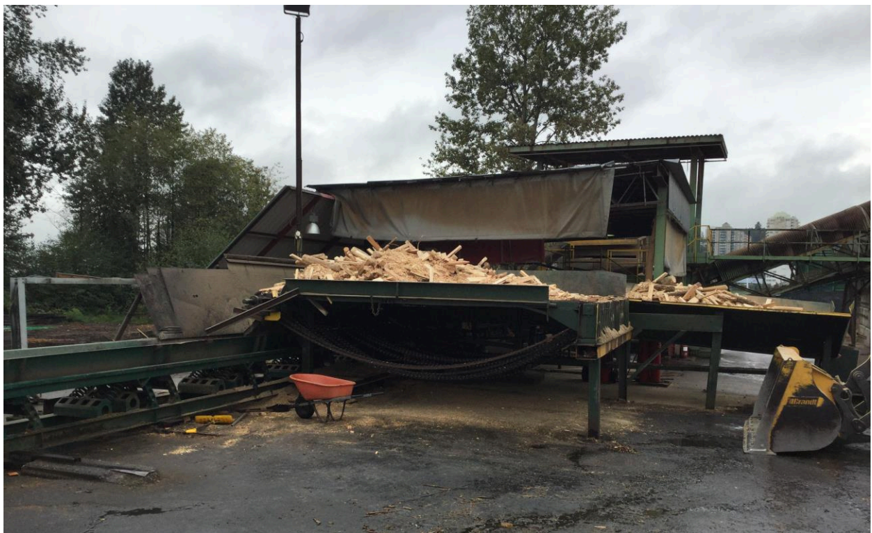
Photo 4. Smallwood Sawmill's wood chipping and conveyer system.
