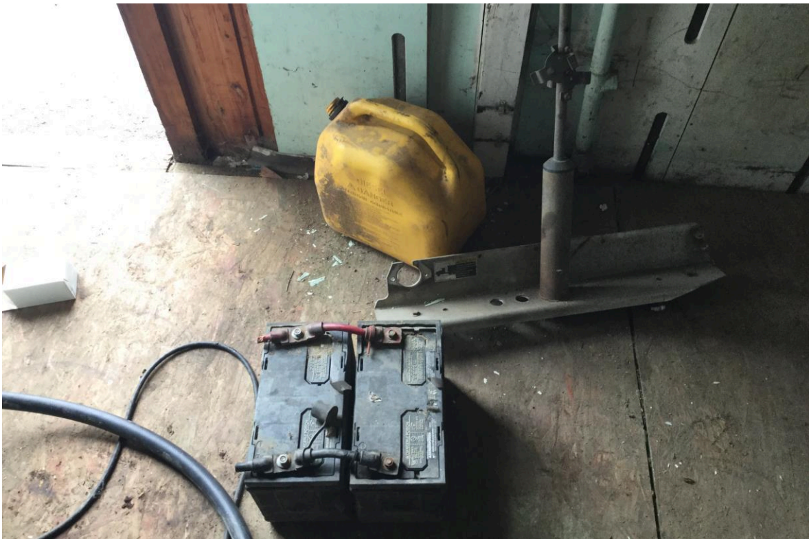
Photo 10. An open diesel fuel jerry can in the AST storage shed.
