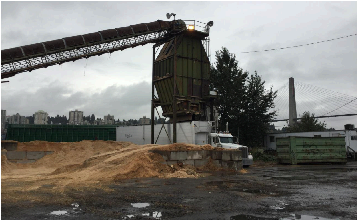
Photo 5. Wood chip loading area, facing north.
