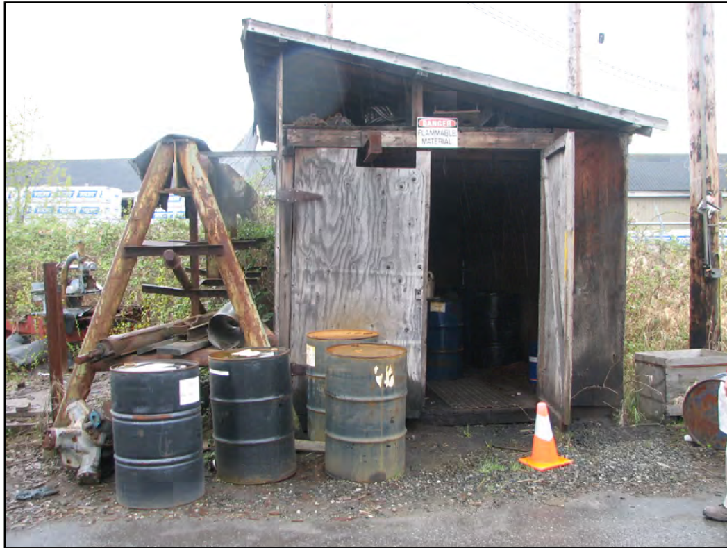
PHOTO 3: Parcel A - Looking southeast at the oil storage shed.
