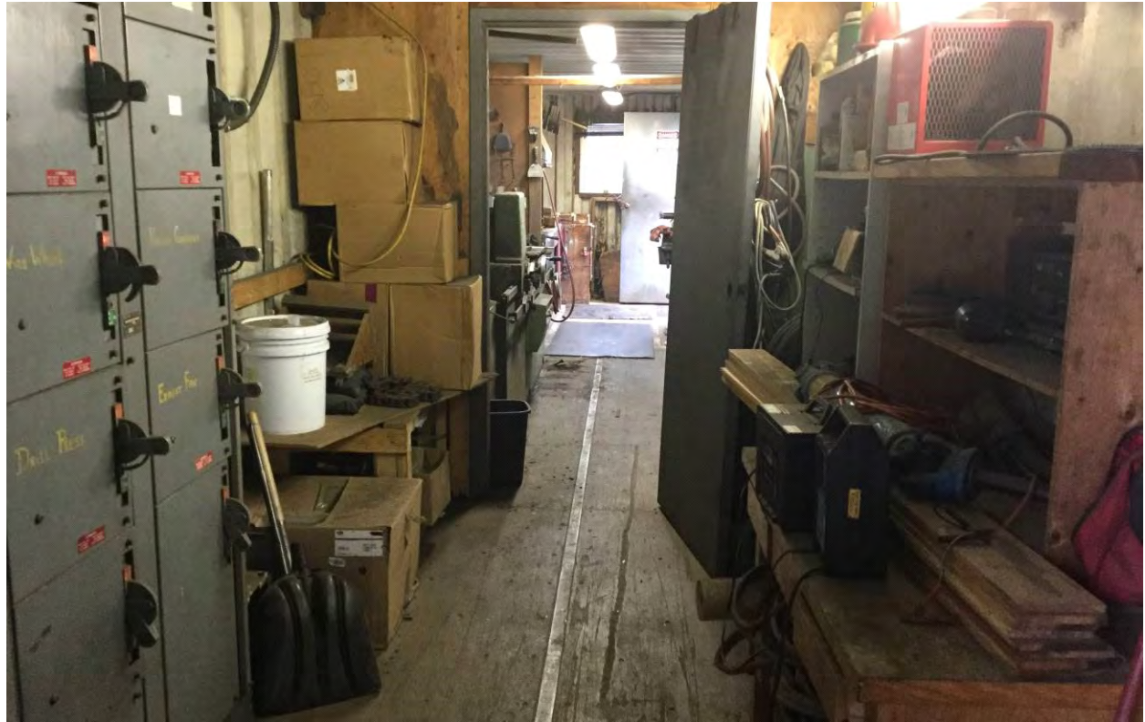
Photo 3. Maintenance and storage room near the wood chipper in Parcel A.
