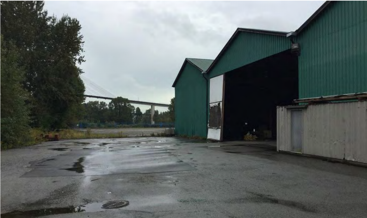
Photo 16. View of the northwest side of the warehouse building and evidence of ground repairs.
