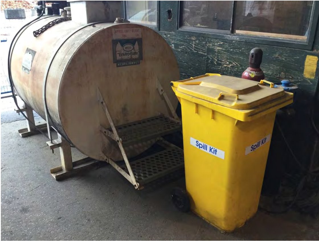
Photo 15. A second AST located at the south end of the distribution warehouse. This tank is double-walled and stores diesel fuel for Panabode's forklift. The tank has only been present for 1 year.
