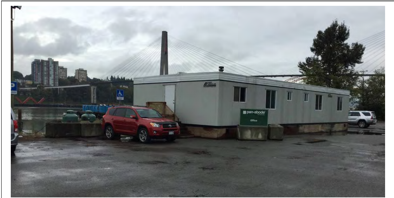
Photo 19. Newly added Panabode office building along northwest edge of the Site, facing north.
