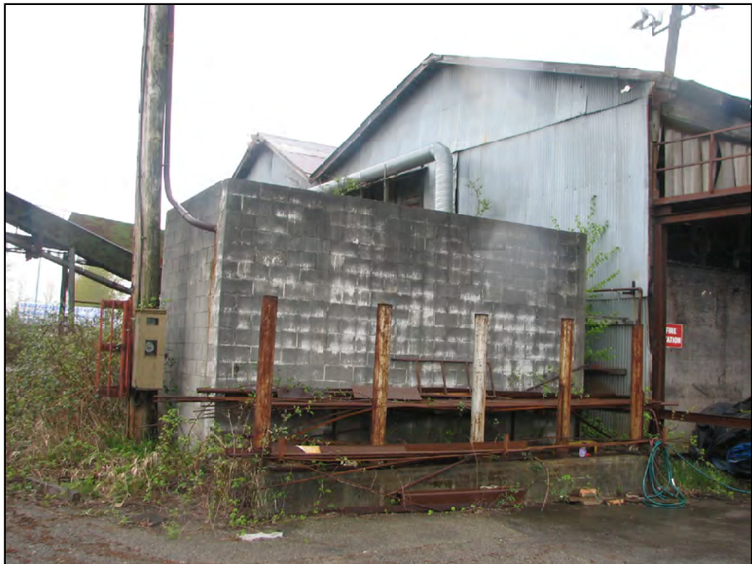
PHOTO 19: Parcel A - Mill Electrical Building.
