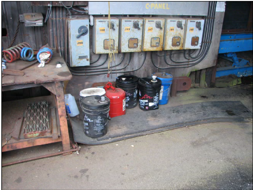
PHOTO 16: Parcel A - View of chemical storage - oil.
