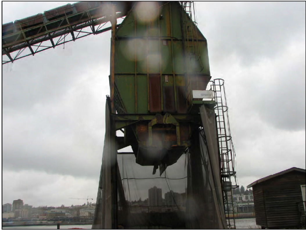
PHOTO 12: View of chip fuel bunker, off-site.
