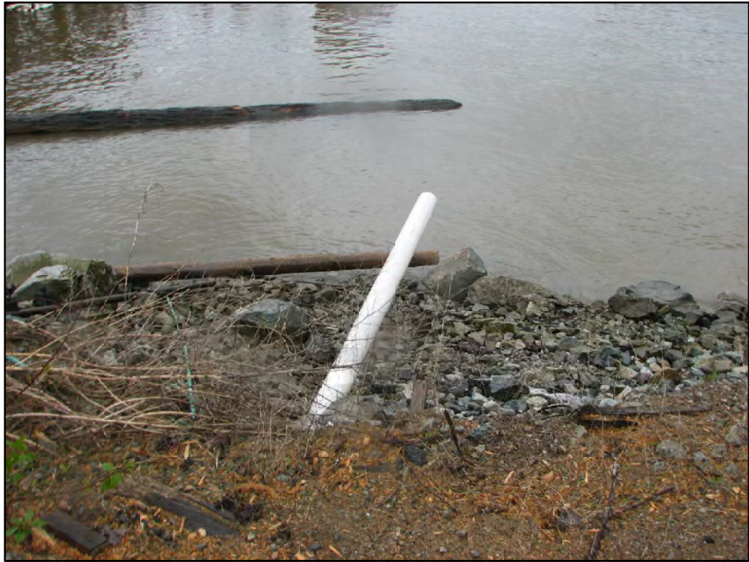
PHOTO 17: Off-site drain outfall on the bank of the Fraser River.
