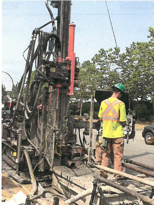
Photograph 1: SPT Hammer on top of AW subassembly at Borehole BH15-04
