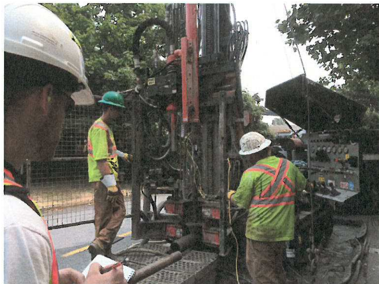
Photograph 2: SPT Hammer on top of NW subassembly at Borehole BH15-14
