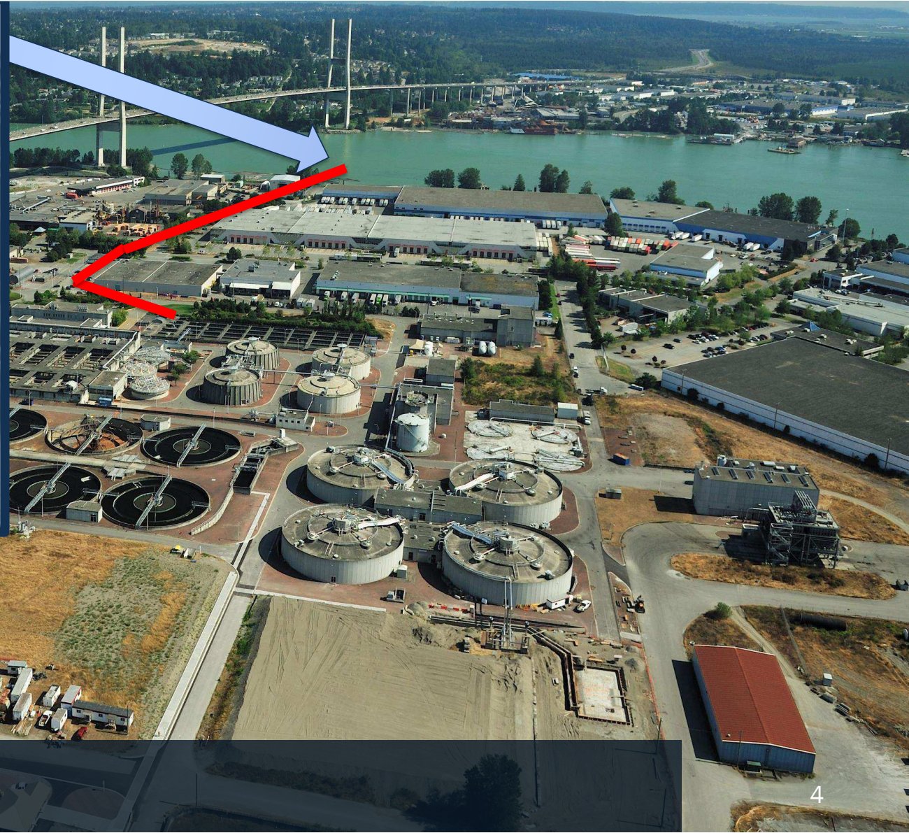
The Existing Outfall
