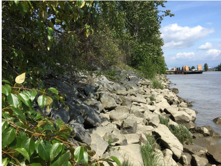
Photo 1: Foreshore of Property consisting primarily of rip rap
